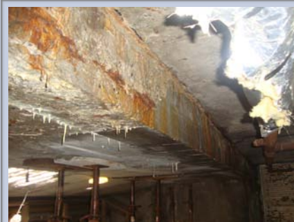
Right: Ramp beam cracking, signs of leakage, and concrete deterioration
