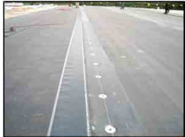
Single ply membrane system secured using fasteners.
